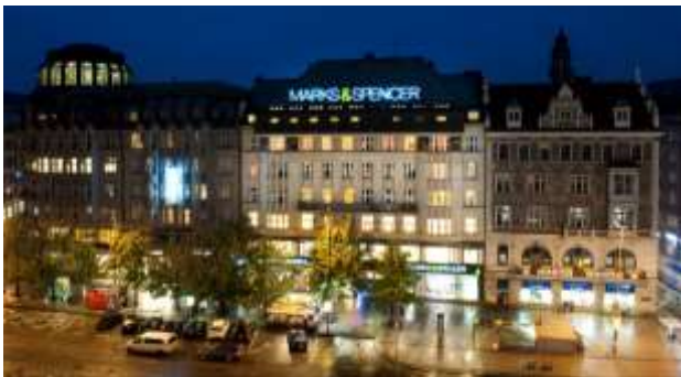
Multifunctional building Melantrich, Praha, Czech Republic
