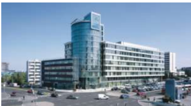
Administrative building Trianon, Praha, Czech Republic
