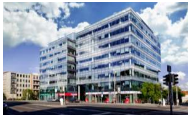
Administrative building Park One, Bratislava, Slovakia
