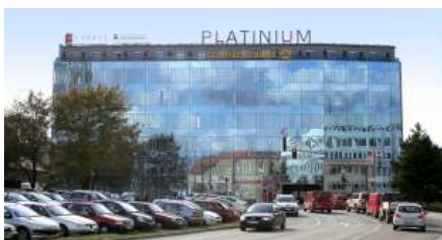
Administrative building Platinum, Brno, Czech Republic
