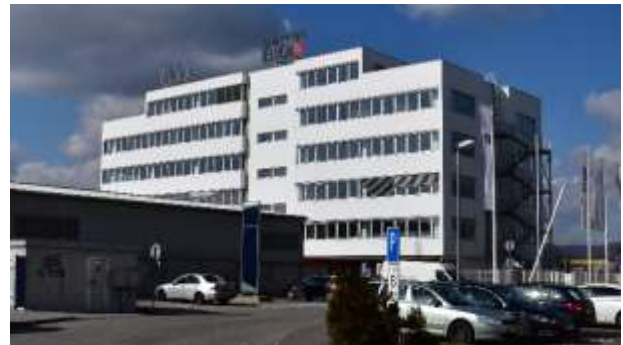
Administrative; Office Box building, Bratislava, Slovakia
